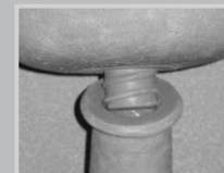
Screw the basin into the pedestal
